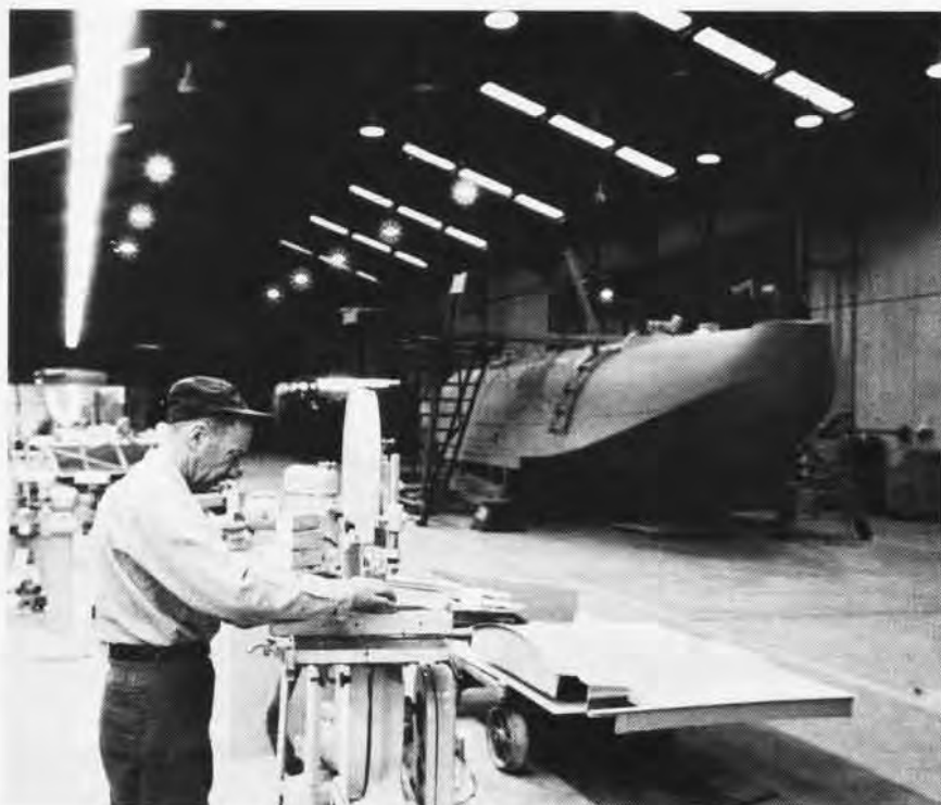
ADR1 Edward Turner (left) makes braces for the NC-4 (hull in background). Below, Harvey Napier, machinist, manufactures small parts for the flying boat. Several of the original parts were lost or broken and had to be made. E. J. Thomas (bottom) directs a crane in fitting the center wing.
