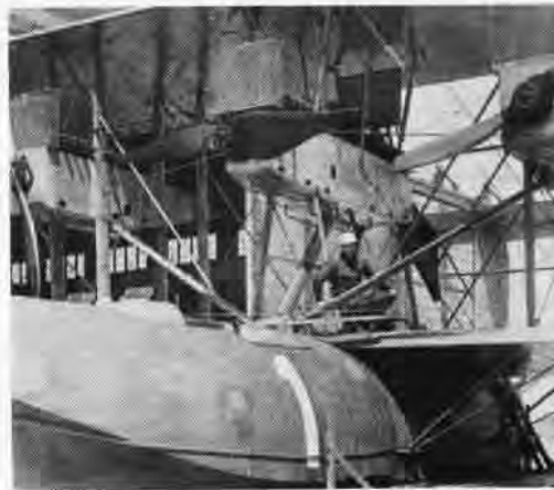
CAUGHT by storm, the NC-1 was battered (above) for three days. Later repaired, it was configured in a 4-engine arrangement similar to the other seaplanes, NC-3 and -4.
