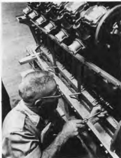
Albert Griffith (above), who recently retired after a career of 30 years at the Smithsonian Institution, works on one of the four Liberty V-12 engines. Griffith did most of the engine restoration work. It takes most of the Silver Hill crew (right) to turn over a wing panel in order to paint other side.
