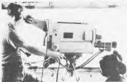
Four cameras, strategically located, zero in on an approaching aircraft. Pictures are fed to PLAT tape in control unit, opposite, from maneuverable camera, at side of flight deck, above, and from two center-line cameras equipped with cross hairs on lens. Fourth camera records time, date, speed and wind velocity.
