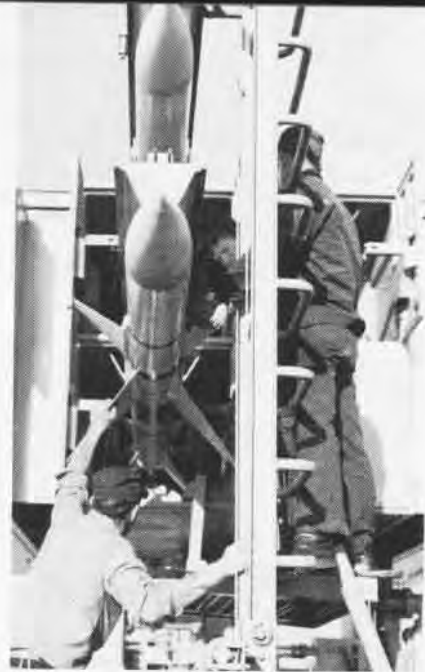
Gunner's mates install test missiles in USS Okinawa's missile launcher, left and above. Below, fire control technician operates the director illuminator during tests.
