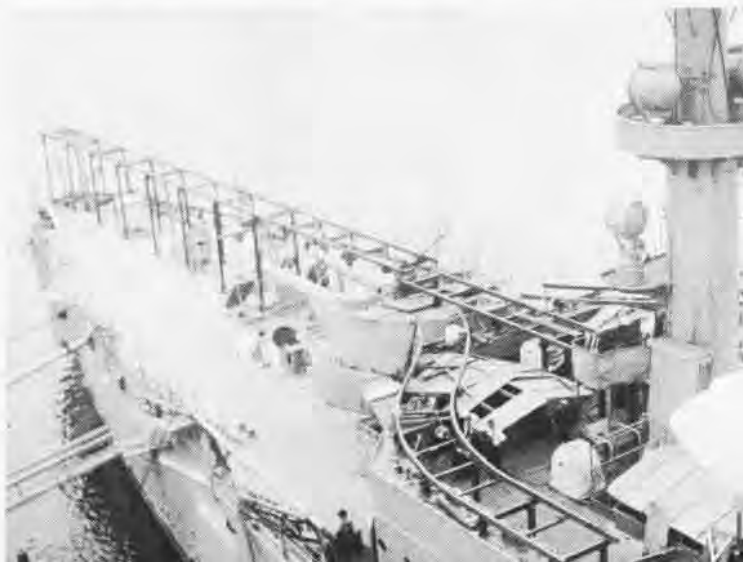
North Carolina, right, in the process of being outfitted with a new catapault, May 1916. Two months later, Lieutenant Chevalier was launched in the AB-3, while the ship was underway.
