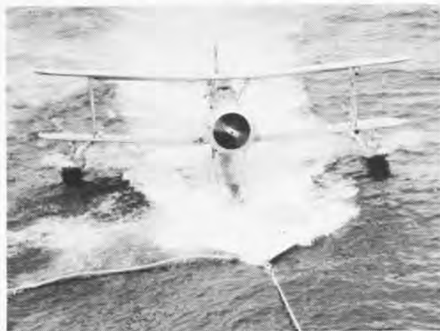
O2U prepares to launch from West Virginia in 1930, using turret-top P-4 powder catapult. An SOC , below, during a CAST recovery.
