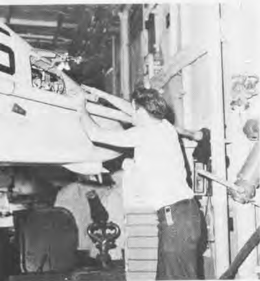
A maintenance man's difficulties are frequently added to by tight working spaces.
