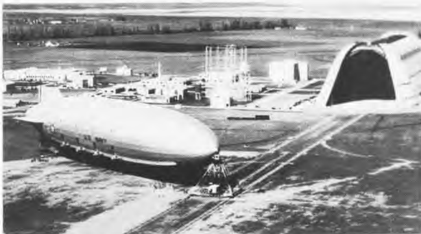
NAS Moffett Field's helium storage plant and airship hangar stand behind USS Macon (ZRS-5) as she is prepared for a training flight from the station's movable short mooring mast.
