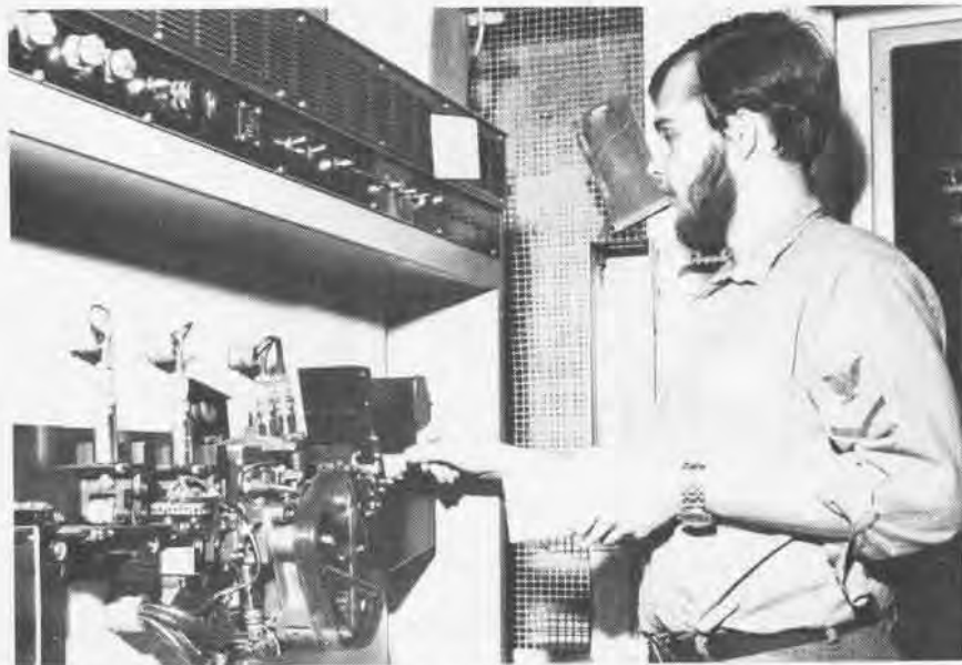
DP3 Kenneth Bachman feeds punch cards to the CRPI (card read, punch, interpret) unit in Kennedy's automated data processing center. Information is then stored on magnetic tape.
