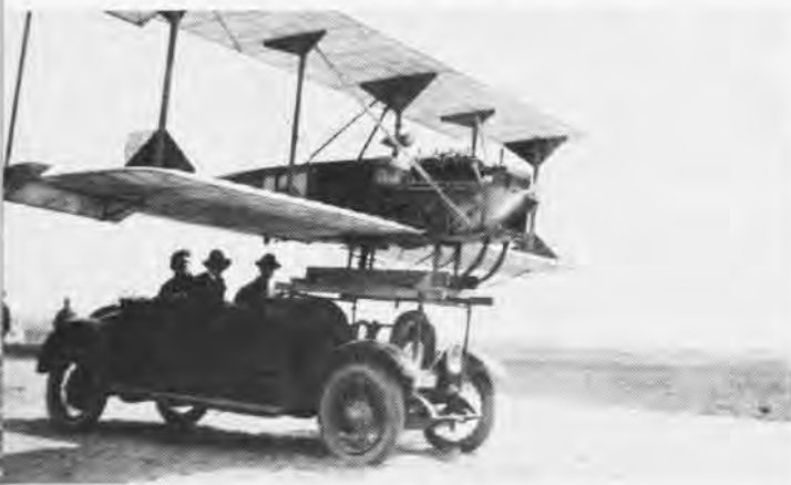
Right, billed as "The world's first guided missile," N2C-2 is put through its paces by VJ-3 sometime during the late Thirties. Marmon car is used as the test vehicle for Sperry Flying Bomb. Below right, TDR-1 over Naval Aircraft Factory.
