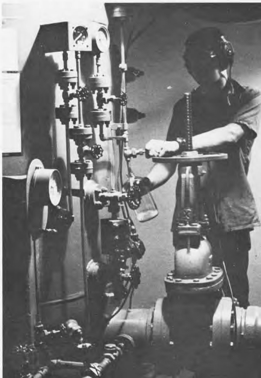
V-4 has several aircraft refueling stations located on the flight deck, above. Fuel samples are taken regularly to ensure quality of avgas, below.
