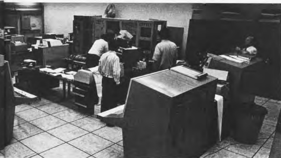
Future tactical support center watch officers will sit at main control consoles such as the one at center above. LCDr. Richard Fidler adjusts an AN/UYK-20 prototype mini-computer, above; in the foreground is the UYK-7 main TSC computer. Engineers work on a computer tape unit, far left. Equipment abounds in the TSC work area where technicians work with and check software programs, left.
