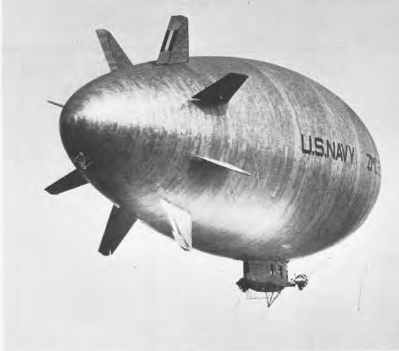
Unusual among Navy airships was 1929 200,000-cu.-ft., twin-engine, metal-clad ZMC-2.
