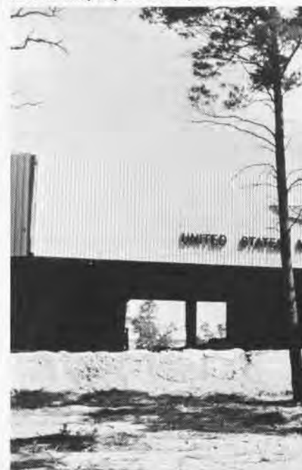
Museum entryway nears completion.
