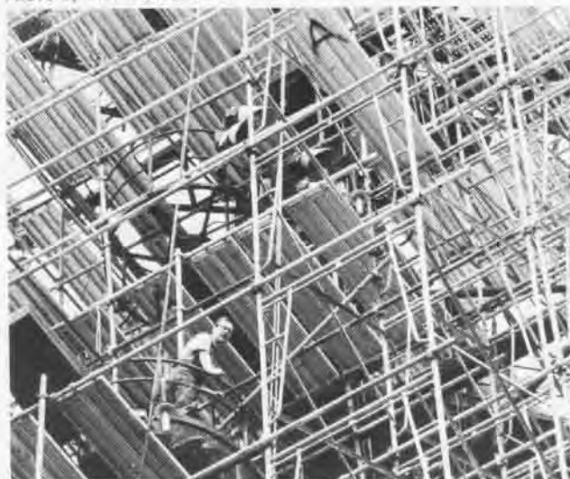
The island on Forrestal had more the look of a high-rise project during her four-month overhaul.
