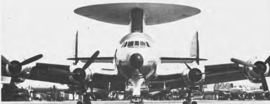
Above, an R7V-1 Constellation bears the markings of the old Military Air Transport Service. Left, a WV-2 airborne early warning version of the Super Constellation sports the "flying saucer" radome in 1956.
