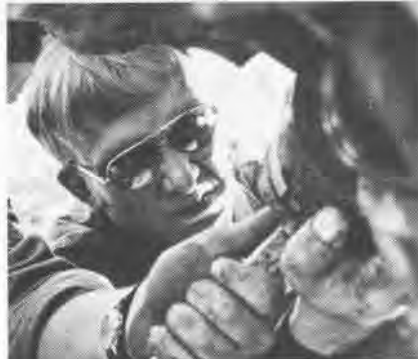
Two aviation structural mechanics change the damper bearing on the flight control of an RH-53D helicopter at NAS Norfolk.
