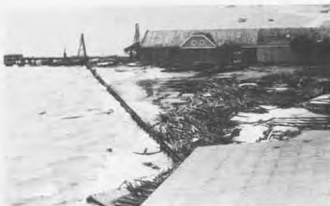
Storm damage at Naval Aeronautic Station, Pensacola in July 1916.
