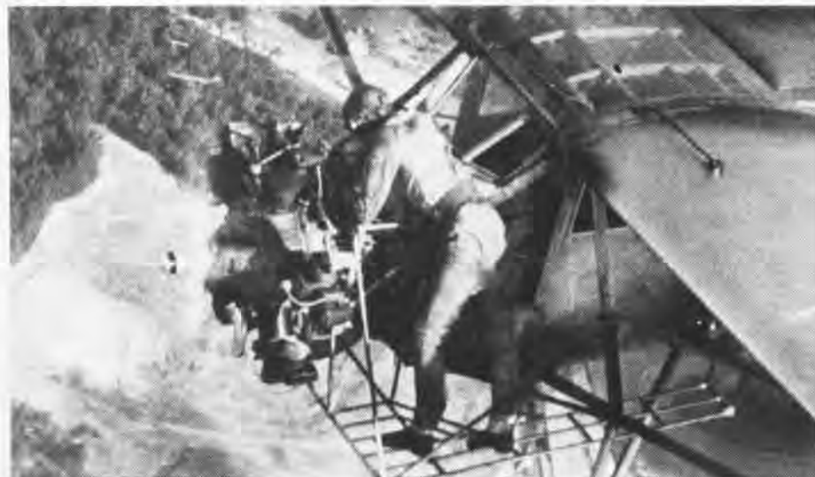
Fred Key services the engine of "Ole Miss" during the record-breaking sustained flight in 1935.
