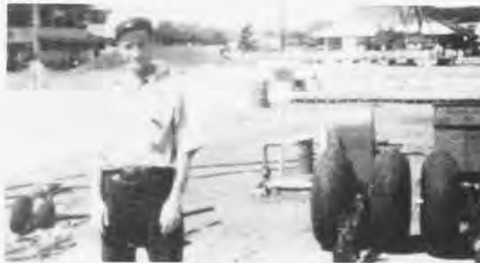
One of VP-21's chief petty officers with PBV beaching gear and barracks under construction in the background, Sangley Point, 1939-40.
