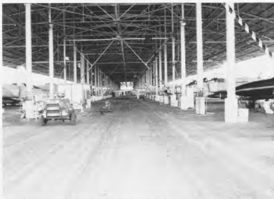
An open view of the maintenance hangar where the preparation of the aircraft takes place. The cover of the facility is painted white to help dissipate the desert heat.
