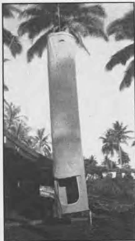
THE PORTABLE TOWER AIDS IN DRYING CHUTES
