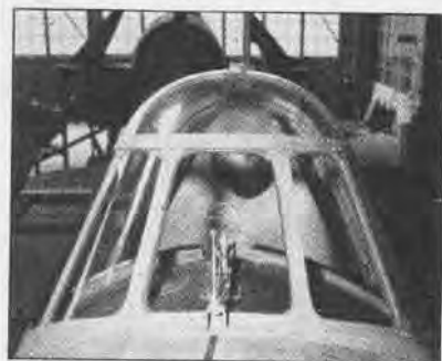
TORPEDO DIRECTOR ATTACHED TO PLANE
