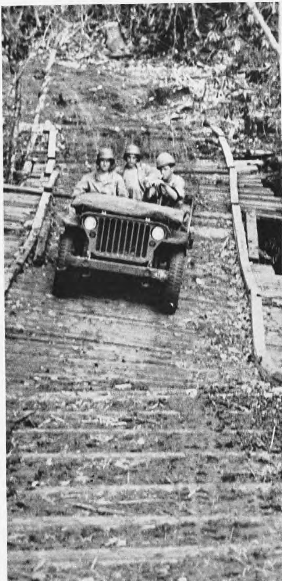
MARINES USED AMPHIBIAN TRACTORS TO PROVIDE FOUNDATIONS FOR THIS GUADALCANAL BRIDGE
