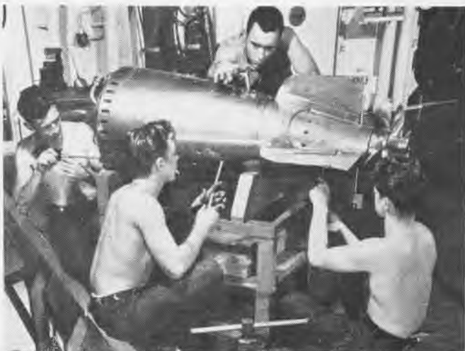
ORDNANCEMEN IN HOLD OF CARRIER ADJUST TORPEDO'S MECHANISM
