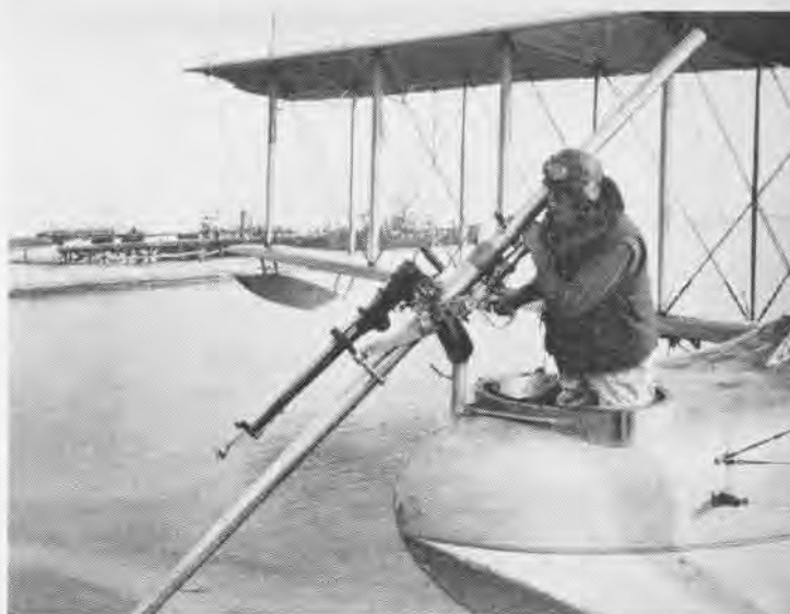
DAVIS gun, intended for attack on submarines, charged through both ends of long barrel instead of having recoil mechanism
