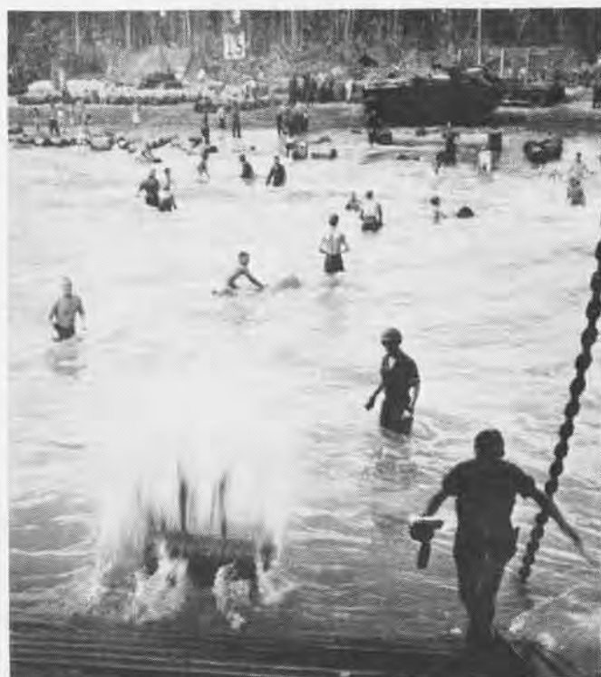
AVIATION gas and Diesel fuel are unloaded at Empress Augusta Bay, Bougainville, by rolling drums down ramp of landing craft
