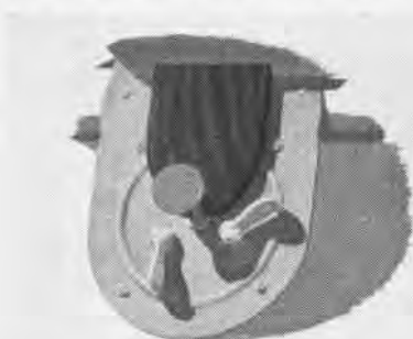
SAFETY GUARD FOR MASTER SWITCH TO IGNITION OF PBY
