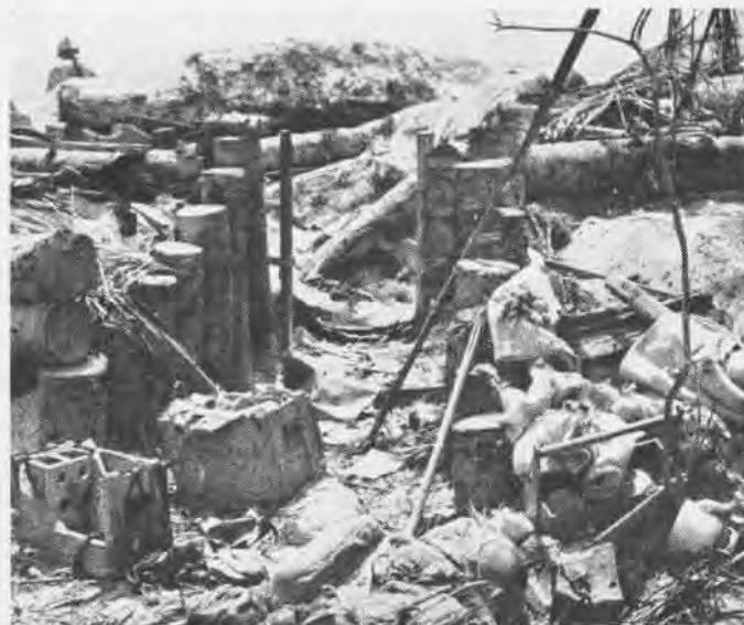
RUINS following direct hit on bomb shelter. Impact of bomb has shattered logs that protected roof, which caved into interior
