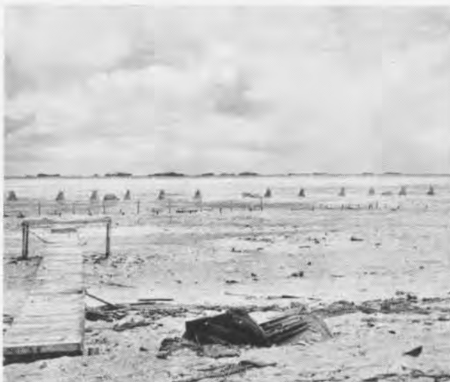
FIRST line of water defense: concrete pyramid boat, tank obstacles. It is low tide and considerably more of base is visible
