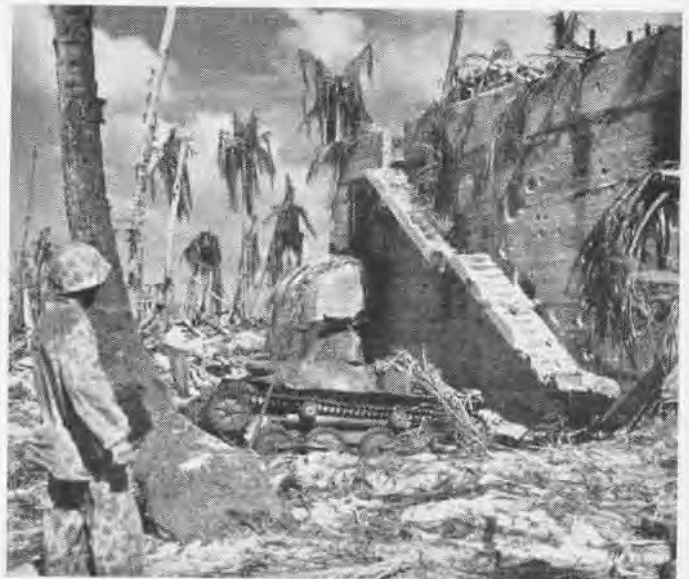
COMMAND post with concrete walls 8 feet thick withstood direct hits from our ships. Roof parapet is reinforced with sandbags
