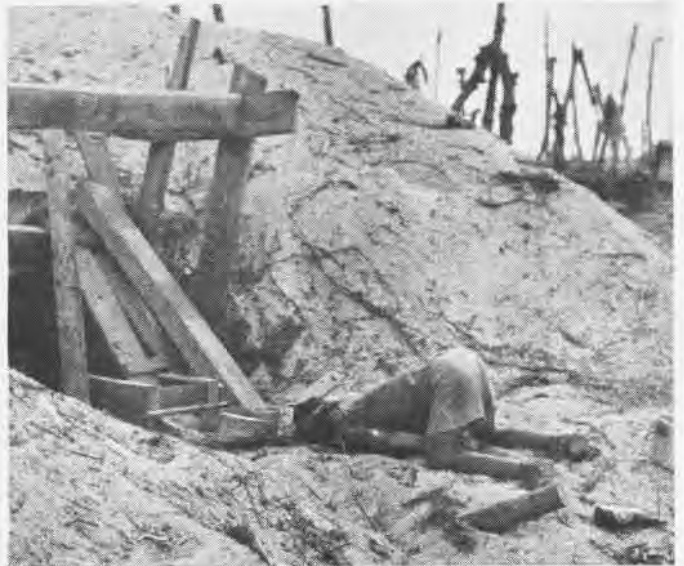
SIZED beams in place of usual coconut logs indicates finished lumber was imported. Jap warrior is nipped seeking safety
