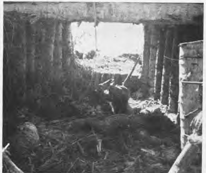
INTERIOR of nest shows two-foot protecting bulwark at farther opening. Notice the thick double row of coconut logs overhead
