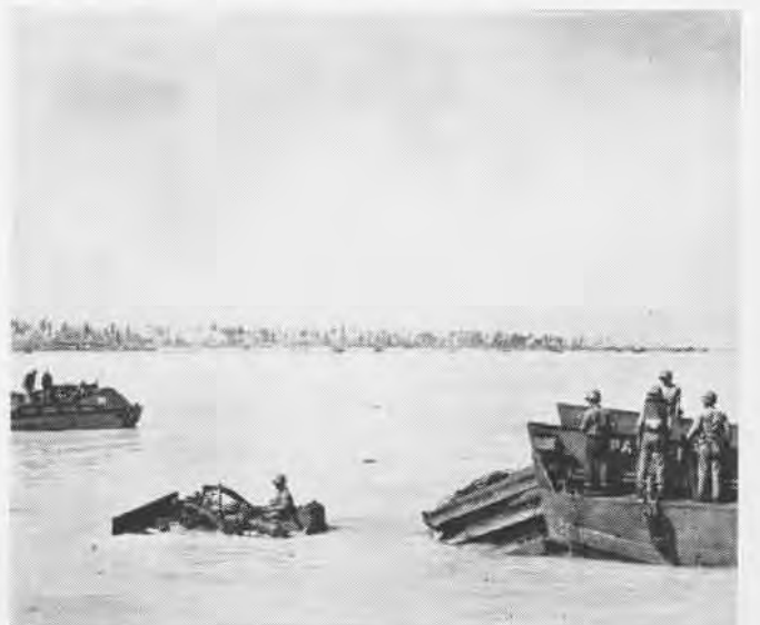
LANDING boat on reef edge with bulldozer in water waist deep. Maze of water obstructions made Marine landing longer process
