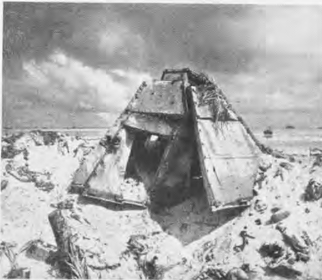
STEEL command post is mobile type brought to Bititu in sections and bolted at corners. Jap inside suggests size of pillbox
