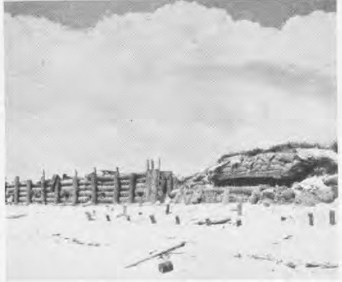
COCONUT log sea wall with gunport located at right, concealing Jap defenders. In front is barbed wire entanglement
