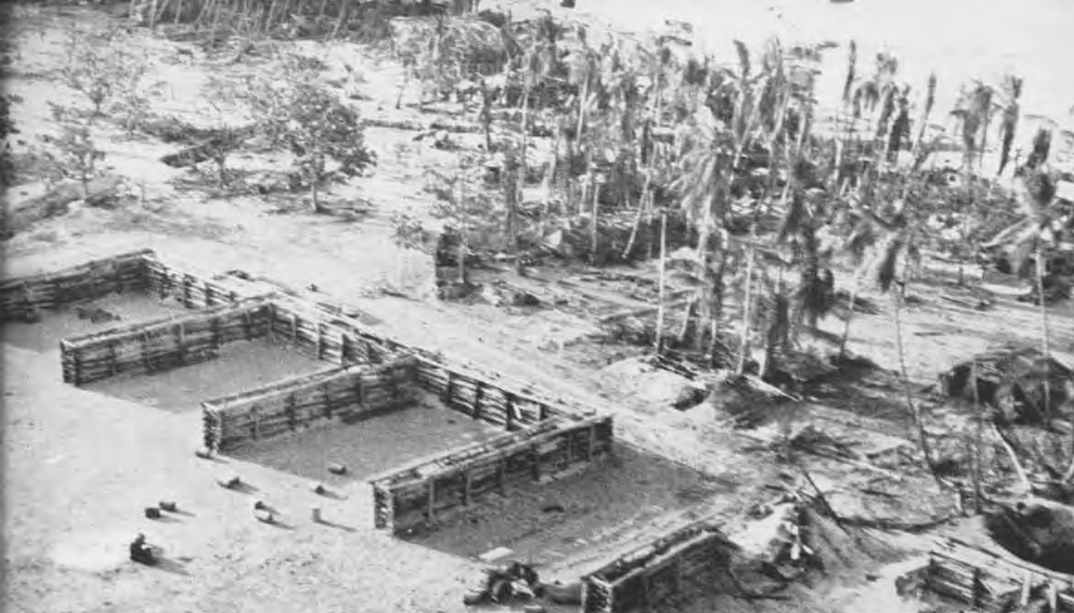
COCONUT LOG AND CORAL REVETMENTS. THERE IS NO SHELTER OVERHEAD. PURPOSE IS TO PROTECT PLANES FROM FRAGMENTATION BOMBS
