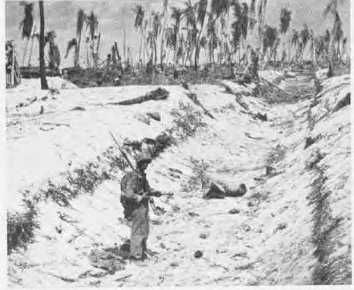
TANK trap's dimensions can be gauged by comparison with Marine standing there. Traps are designed to slow, not stop, tanks
