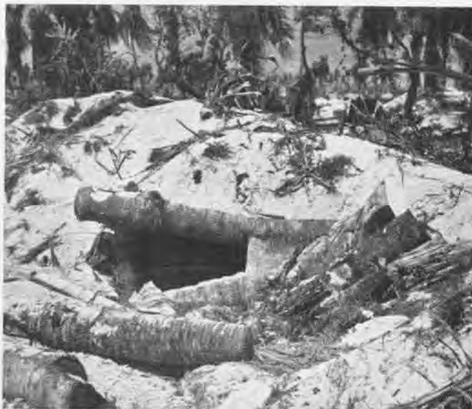
MACHINE GUN nest built with coconut logs and sandbags covered with loose coral. Nest is designed to protect gunnery crew
