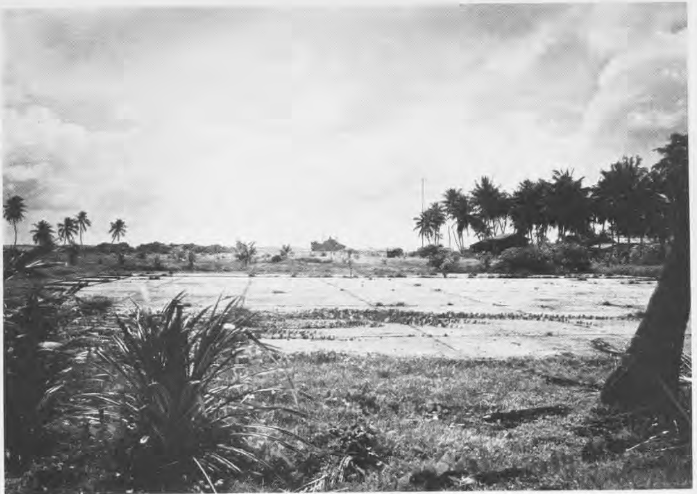
Hangar foundation of concrete was constructed near ramp leading to the lagoon, apparently to protect seaplanes. Size of proposed
