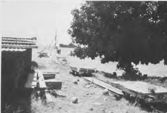
Pier runs out to deep water in lagoon. Narrow gauge railway was used for unloading Jap freighters bringing in building supplies
