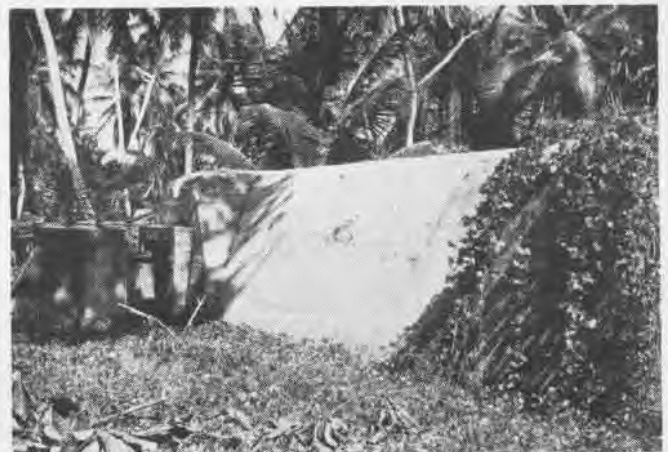
Concrete shelters are of standard design, with thick walls and iron door at center. Firing ports may be provided in both side walls
