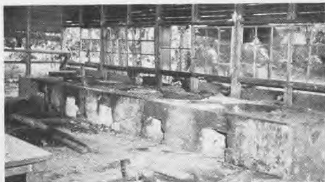
INSTEAD OF CHIMNEYS FOR OPEN OVENS, KITCHEN IS VENTED BY LOUVERS
