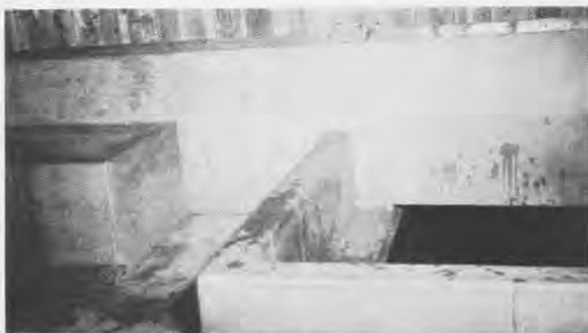
CONCRETE TUBS WITH RUNNING HOT WATER PROVIDE LUXURY OF A BATH
