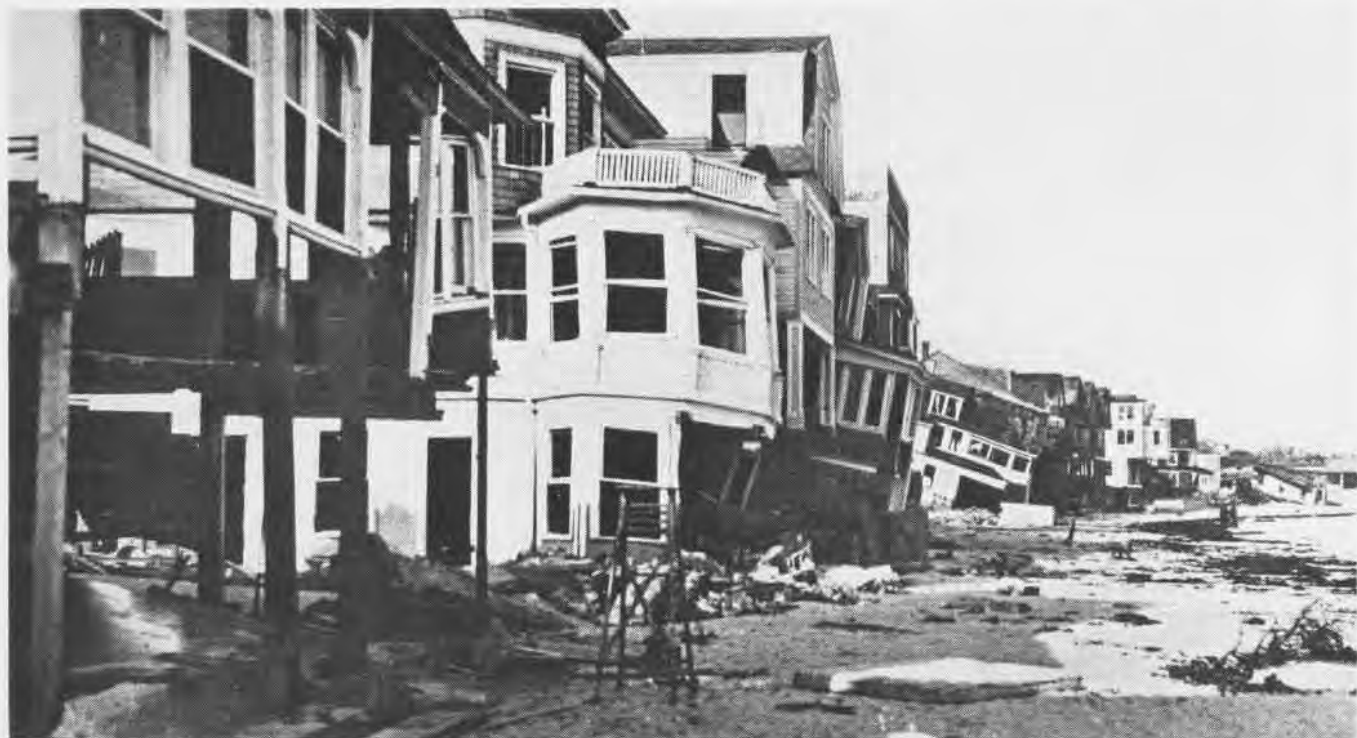
BATTERED BEACH AT NEW LONDON, CONN., REVEALS SOME OF HEAVY DAMAGE INFLICTED ON NEW ENGLAND COAST IN HURRICANE OF SEPTEMBER, 1938
