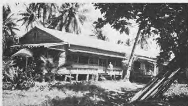
HEADQUARTERS BUILDING RESTS ON FOUNDATION OF COCONUT LOG PILING
