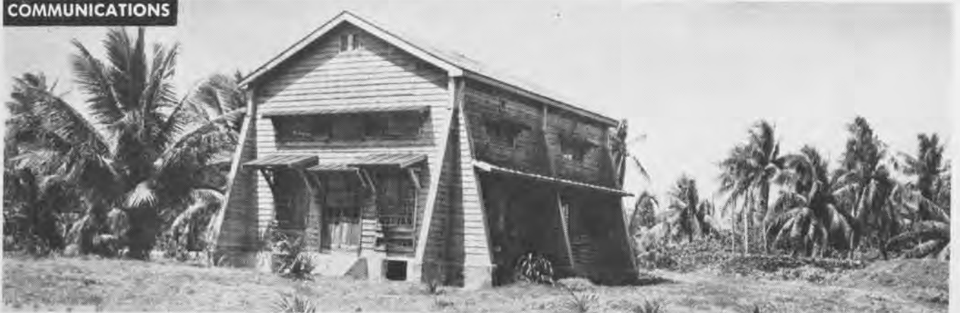
Overhanging eaves and buttresses made this building appear larger in aerial photographs that it actually was. It was built to house
