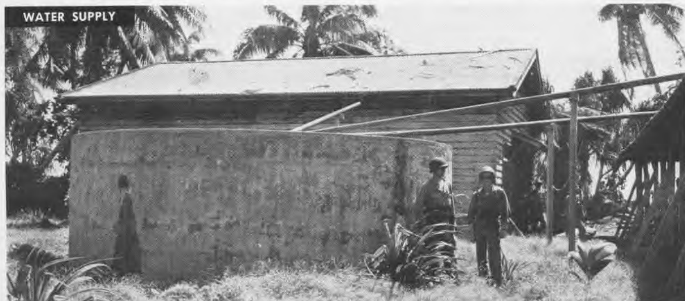
WATER SUPPLY RAIN WATER IS THE ONLY AVAILABLE SUPPLY FOR DRINKING, COOKING, WASHING. IT IS COLLECTED AND STORED IN CONCRETE TANKS, CISTERNS
