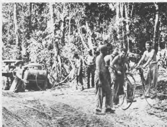
5 Sometimes the crystalline coral was so tough the Seabee's bulldozers could not shove it aside and dynamite crews had to be called in to blast it out. Here pneumatic hammers drill holes for the dynamite to be tamped in and work of leveling continued
