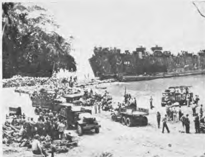
2 Five days later the bulldozers had shoved back enough undergrowth so that supplies and equipment could be landed on the sandy beach and the push into the jungle started. Japs lurked in the interior of the island but they did not seek a showdown
