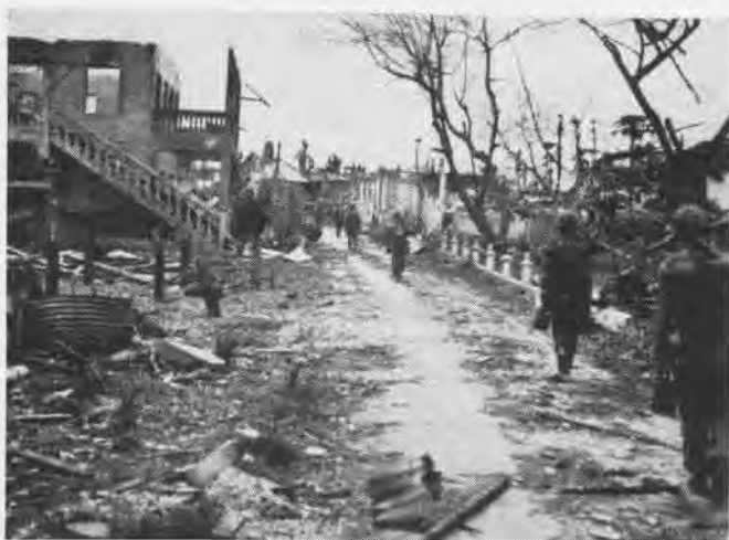
U. S. Marines walk the streets of Agana again after the invasion. A heavy toll was taken of city's structures by U.S. bombardment
