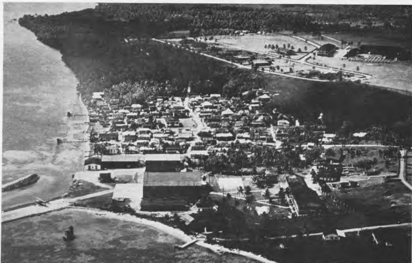
THIS PRE-WAR AIR VIEW OF OROTE PENINSULA, GUAM, SHOWS THE TOWN OF SUMAY, PAN AMERICAN AIRWAYS FACILITIES AND MARINE RESERVATION
