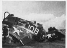
tle, but got no response from his engine. The Bearcat hit 500 feet short of the LSO with the left wing down. The wing tip broke off on impact, and the plane was righted and rolled 300 feet angling across the runway. When it hit a soft area the F8F flipped over and skidded about 35 feet on its back.
