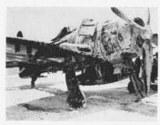
By this time the fire had burned itself out, but the pilot must have been surprised when he looked at the area back of the cockpit. The damage report states that 50 to 75 percent of the underside of the fuselage between the wheel wells and the tail wheel was completely burned away.
